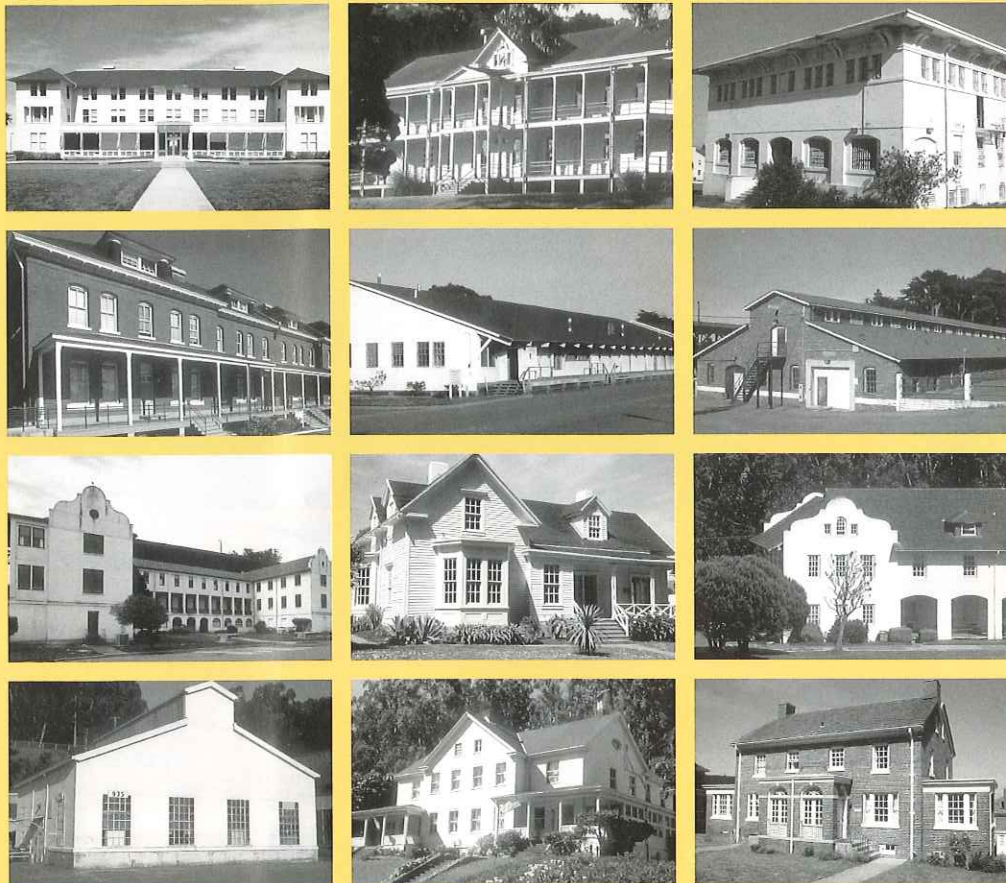
Row One, L to R: Bldg. 1016 (Historic Letterman Hospital), Bldg. 682 (Former Cavalry Barracks), Bldg. 1213 (Fort Scott Stockade) Row Two, L to R: Bldg. 103 (Montgomery St. Barracks), Bldg. 1163 (Letterman Warehouse), Bldg. 667 (Former Cavalry Stables) Row Three, L to R: Bldg. 650 (Stilwell Hall), Bldg. 10 (Funston Avenue Quarters), Bldg. 1217 (Fort Scott Barracks) Row Four, L to R: Bldg. 935 (Former Aero Storehouse), Bldg. 1304 (Kobbe Ave. Quarters), Bldg. 727 (Liggett Ave. Quarters)
